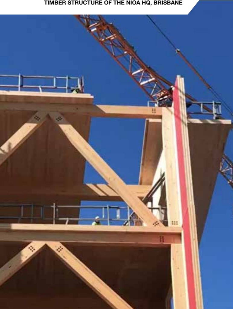
TIMBER STRUCTURE OF THE NIOA HQ, BRISBANE
