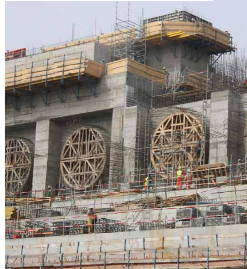
DAM AND HYDROELECTRIC POWER PLANT, NACHTIGAL, CAMEROON
