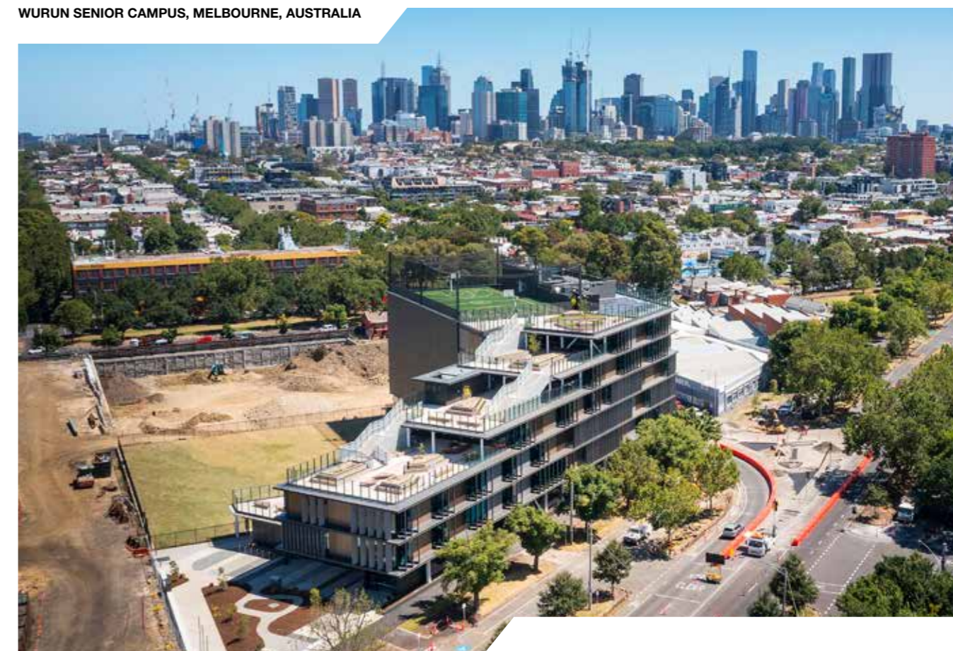
WURUN SENIOR CAMPUS, MELBOURNE, AUSTRALIA
