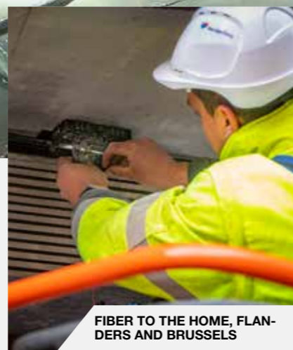
HORIZONTAL DIRECTIONAL DRILLING, ZEEBRUGGE
